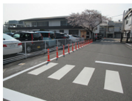
Separating vehicles and pedestrians by installation of soft poles (Kyoto Plant)
