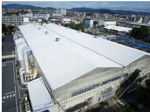
Factory roof after thermal insulation coating
