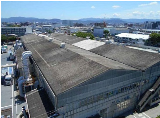
Factory roof before thermal insulation coating
